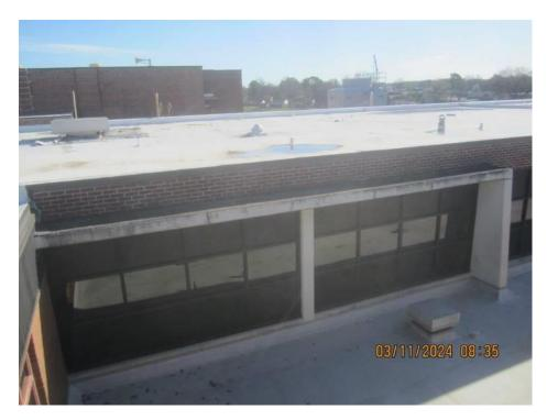
**Item #2** – Contractors are to include the small roof at the classroom wing. This roof shall match the surrounding new roof areas designed with the necessary R-Value and taper to direct moisture and reduce ponding. Install a small gutter system to contain moisture at selected drainage point. Gravel stop to be used at rake edge chosen to direct moisture towards gutter edge. (Attached photo for reference).
